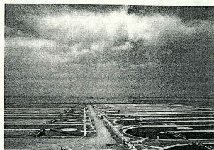
Figure 6-2. Another view of the ponds from the top of the harvest building, showing the harvest pipe system.
