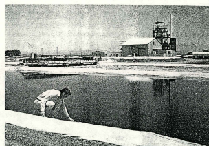
Figure 6-3. Looking across a pond towards the harvest and drying building at Earthrise Farms.
